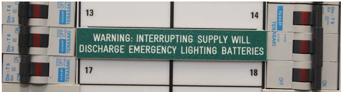
Individual label for each circuit
